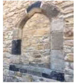
Doorway framework in Mercury House wall
